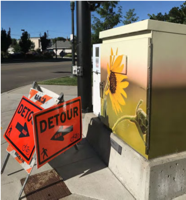
Traffic box with artwork at 13 th St. and River St. showing territoriality.
