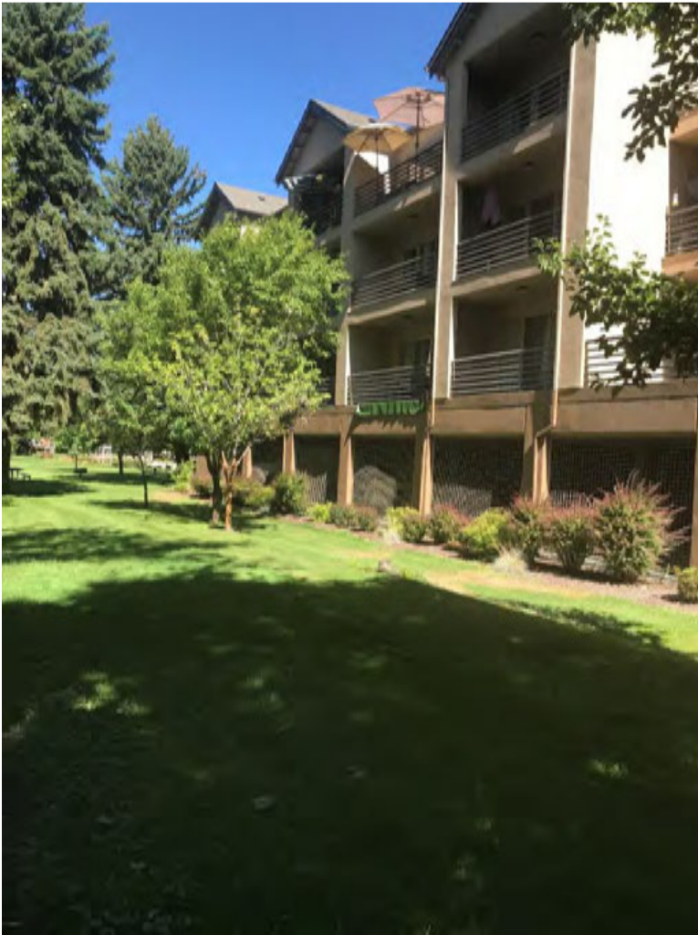
Screens controlling access into the River Walk parking garage. The open grating lets in light and gives visibility.
