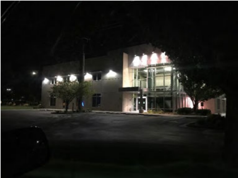
Perimeter lighting at 1649 Shoreline Dr.
