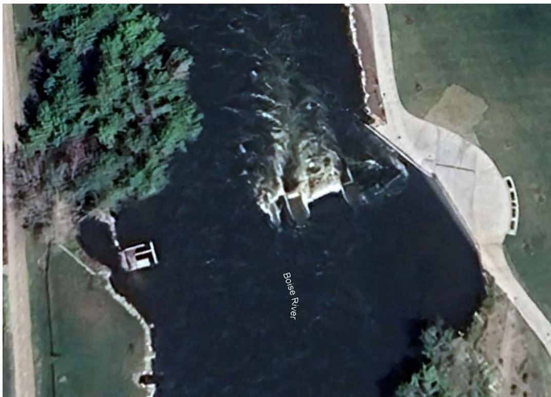
Figure 3. Whitewater Park Phase 2, first feature components at high water.
